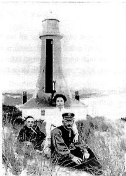
The Braunton Lighthouse The keeper explained to us the regulation numbers of the winds
